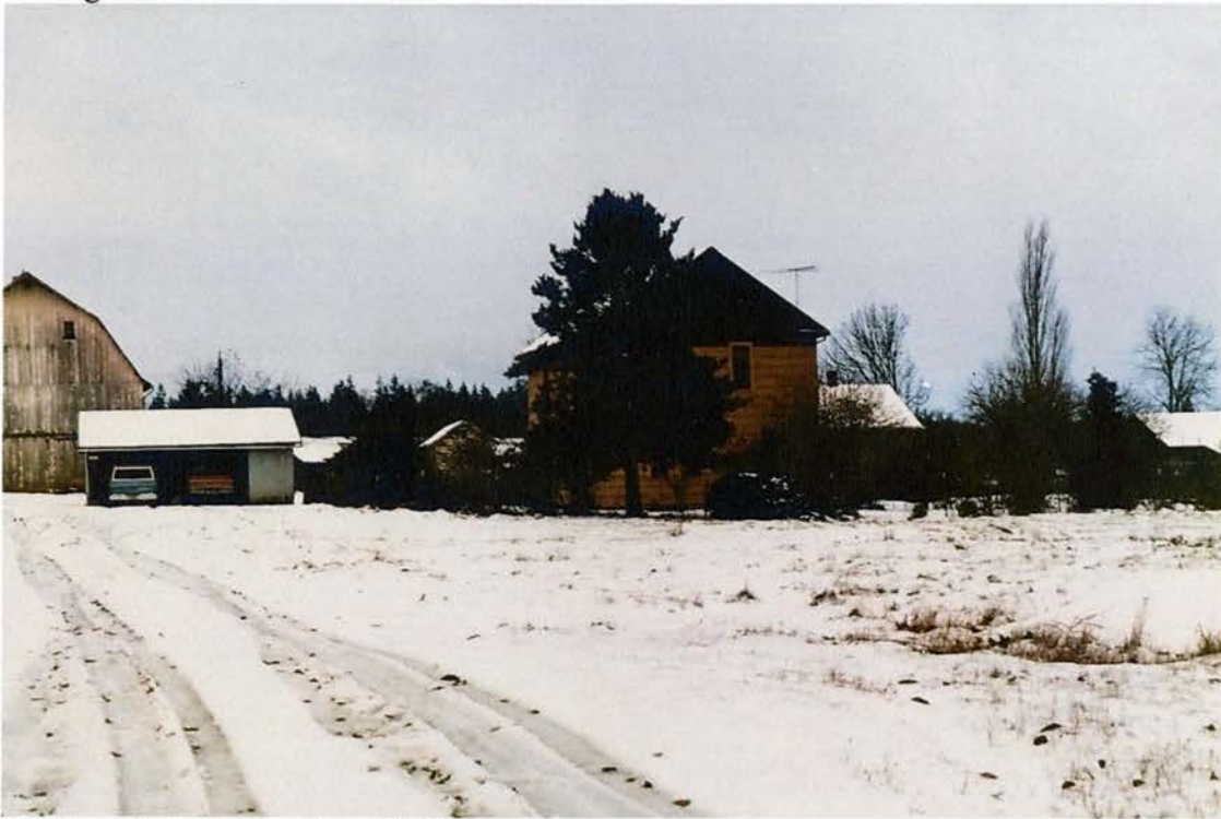
Old Farm house after fire - 1985
