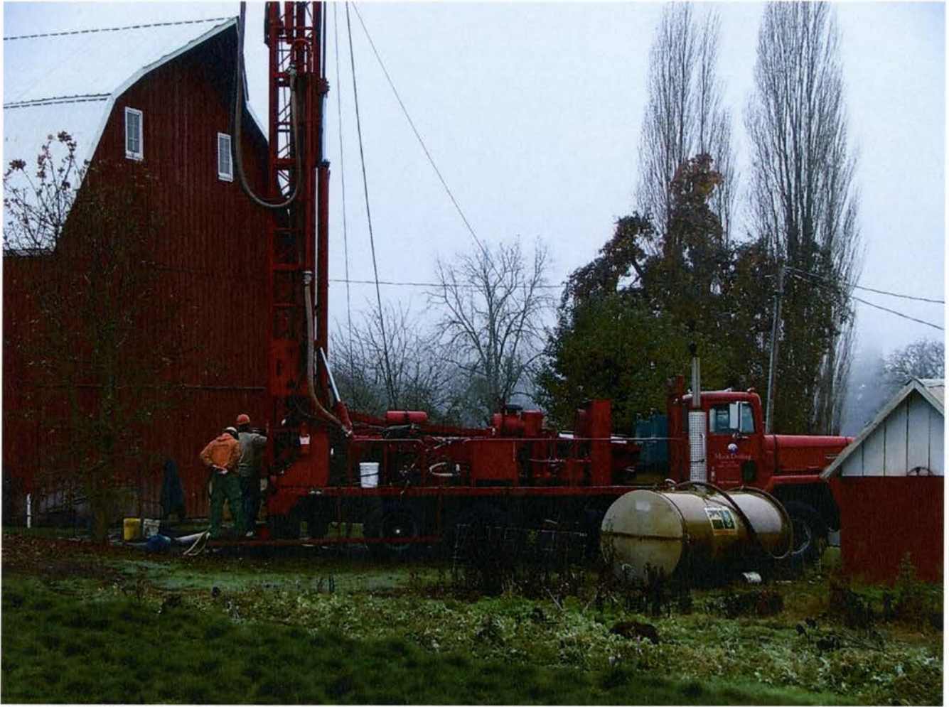
New Well 313 Feet to good water in 2004
