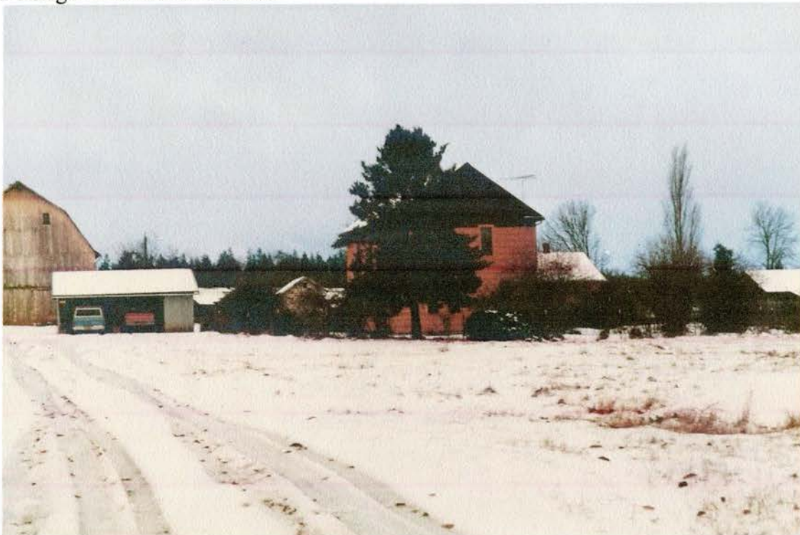
Old Farm house after fire - 1985
