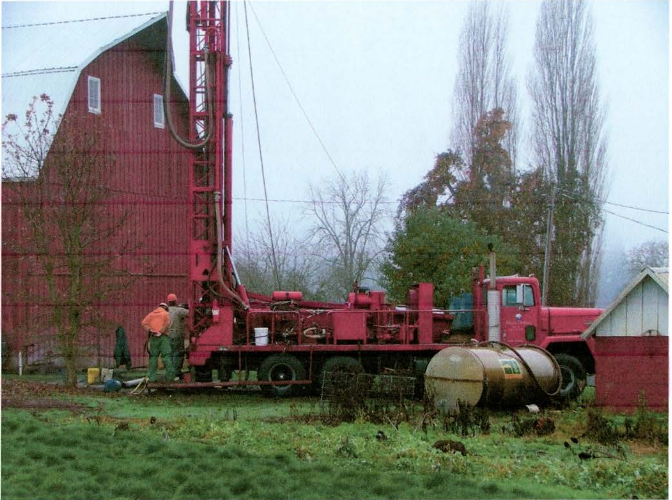
New Well 313 Feet to good water in 2004
