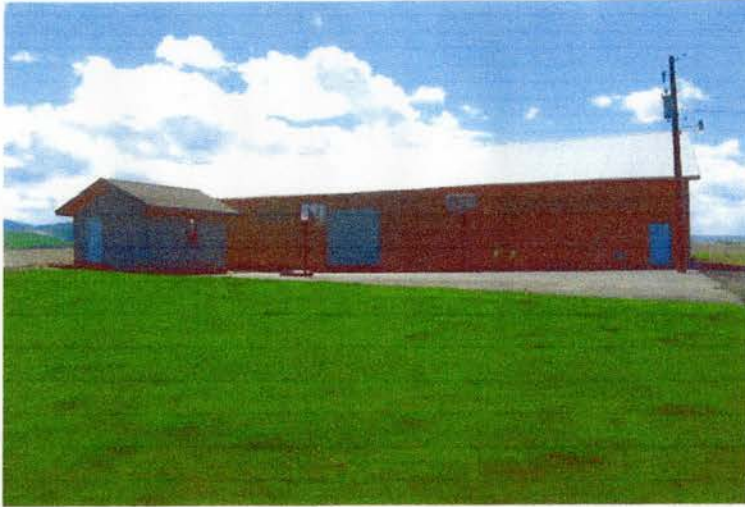
Combine shop with remodeled original bunk house in foreground.
