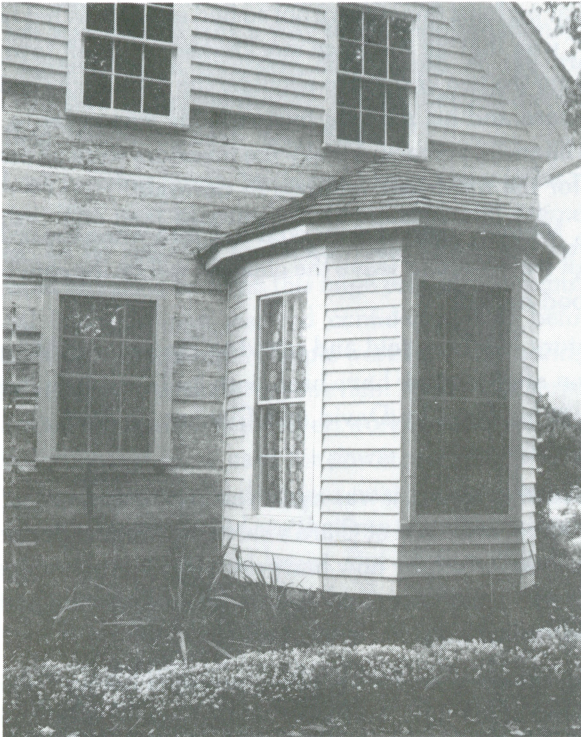
Bay window built by Clara and a hired man during the three year period that David was gone. Neither Clara nor the man understood structural support, and as a result, the east side of the house sagged badly until it was repaired during the restoration in 1982.
